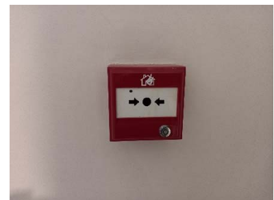
Fire Alarm Manual Station
